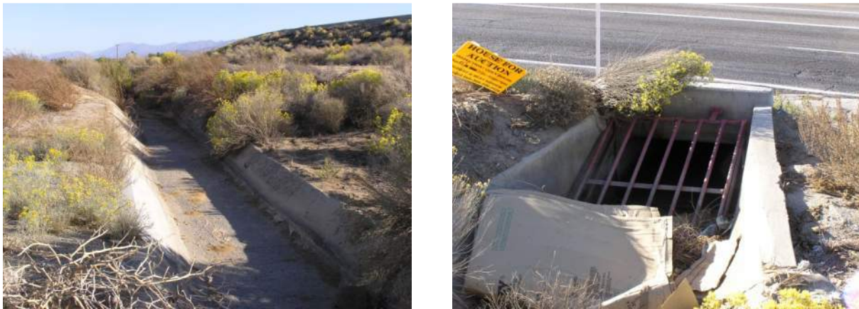
Figure 3-4: Palmdale Ditch & Bar Screen
