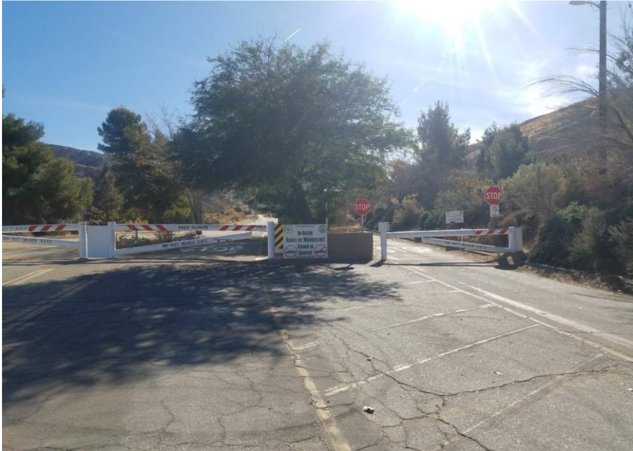
Figure 10-1: Littlerock Reservoir Gated Entry
