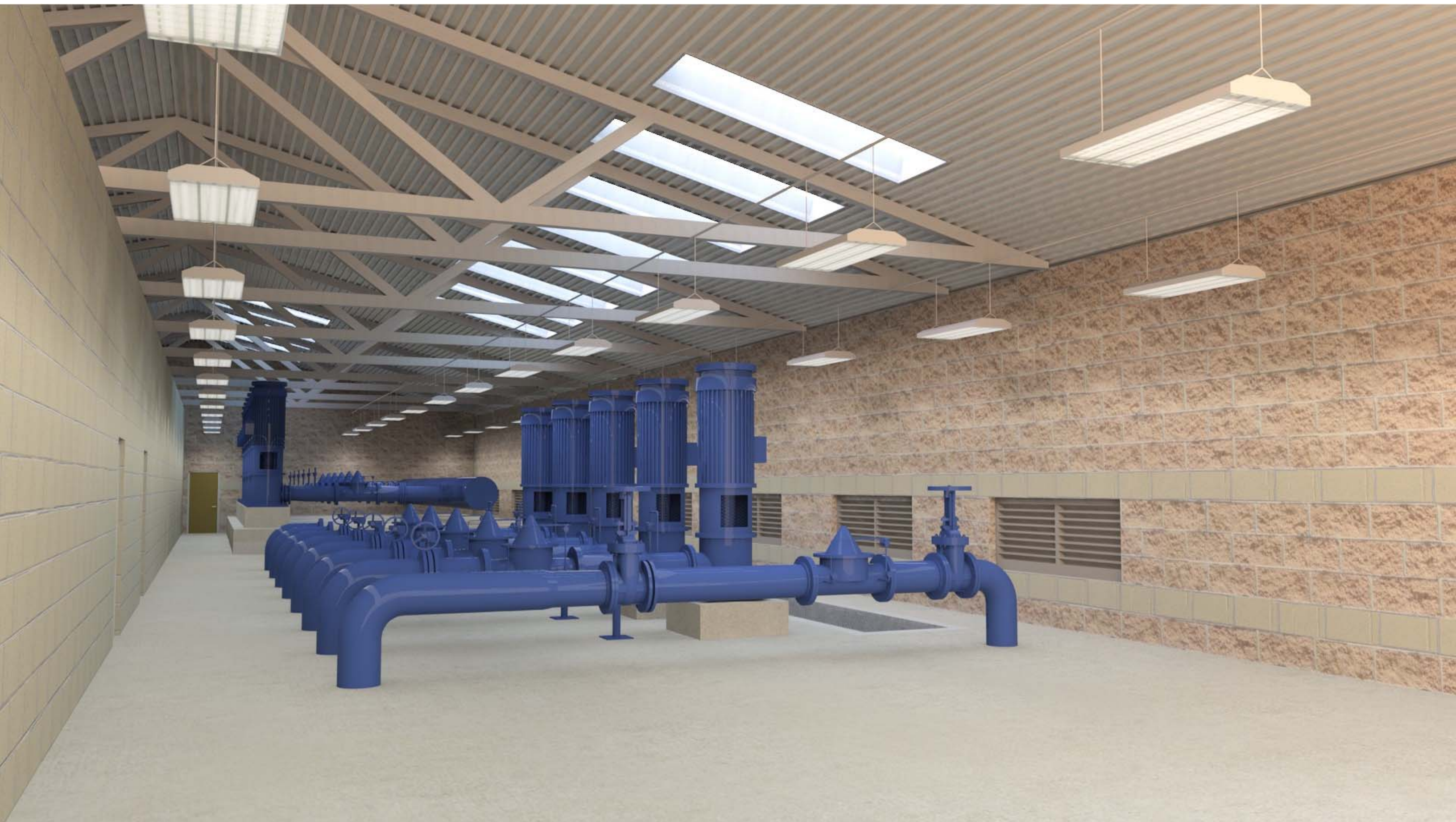
Figure 2: Vertical Turbine Pump Station Rendering
