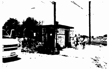
Major Transportation Corridor (Well 20)
