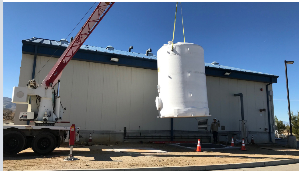
The new saltwater brine tank is installed at the treatment plant.
