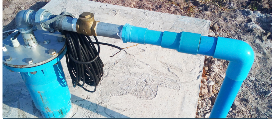
A similar monitoring well will be built for PWD.
