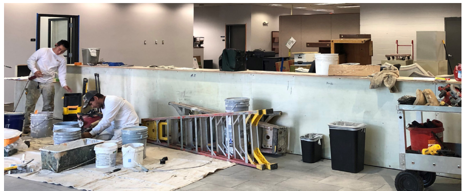
Contractors paint and re-tile the lobby.
