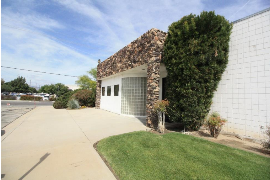
PWD Headquarters, south (primary) façade, view to northwest (ESA April 30, 2018)
