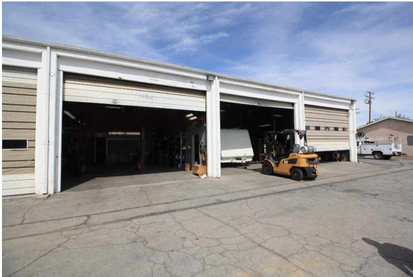
Garage, east (primary) elevation, view to northwest (ESA April 30, 2018)
