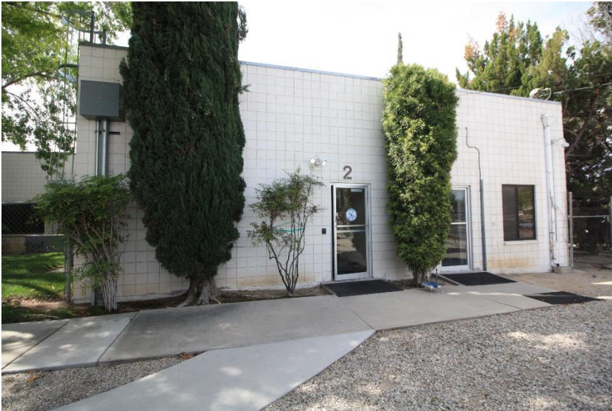
PWD Headquarters, north (rear) elevation, view to south (ESA April 30, 2018)
