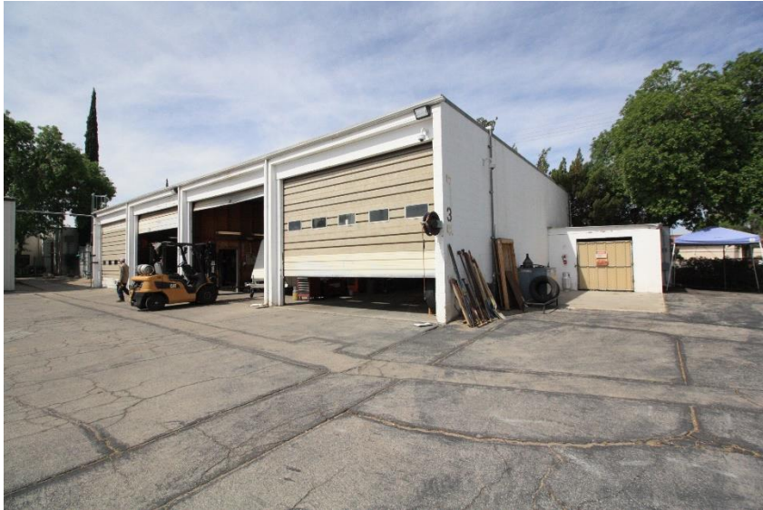
Garage, east (primary) and north elevations, view to southwest (ESA April 30, 2018)
