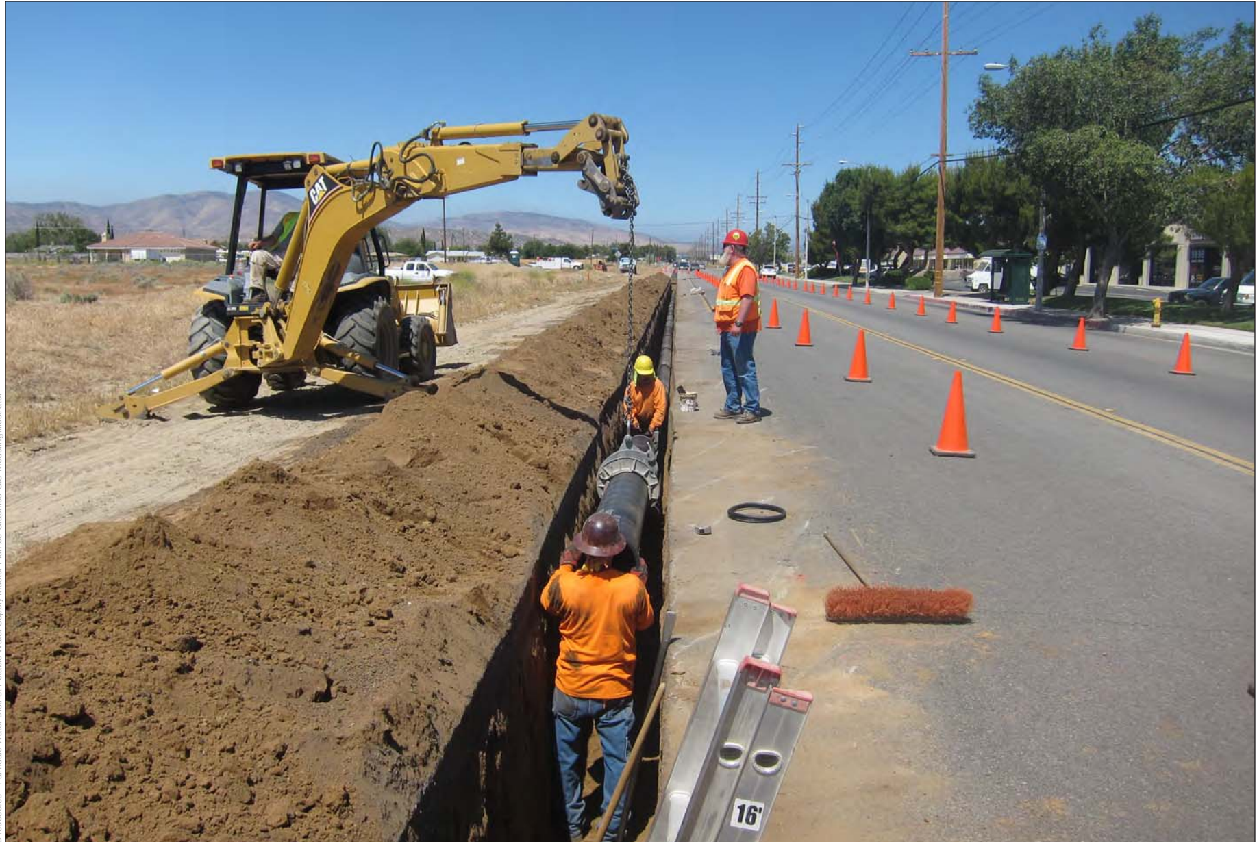
Figure 3.1-3 Replacement of Existing Pipeline within PWD Service Area
