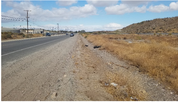
Photo 19. Pipeline along Sierra Highway where it crosses the PWD-maintained Palmdale Ditch.
