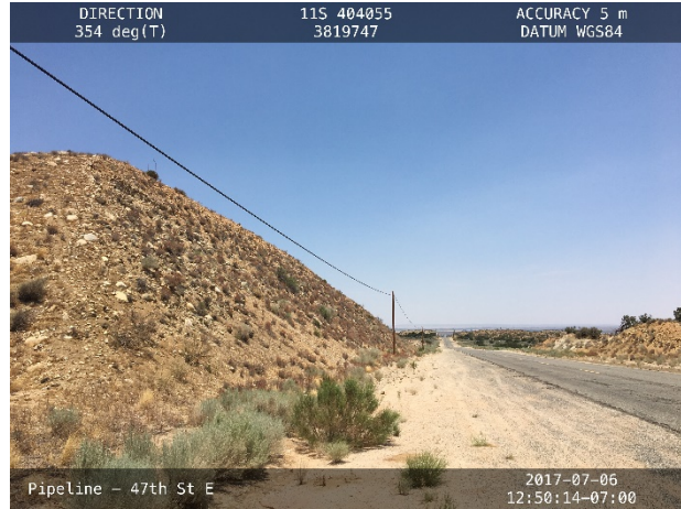
Photo 16. Southern portion of Pipeline along 47 th Street East, sited to the west (left) of 47 th St. East.
