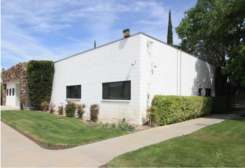
PWD Headquarters, south (primary) elevation and portion of the west elevation, view to northwest (ESA April 30, 2018)
