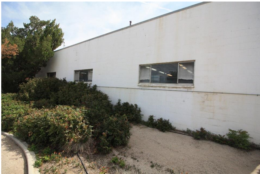
Garage, west (rear) elevation, view to northeast (ESA April 30, 2018)
