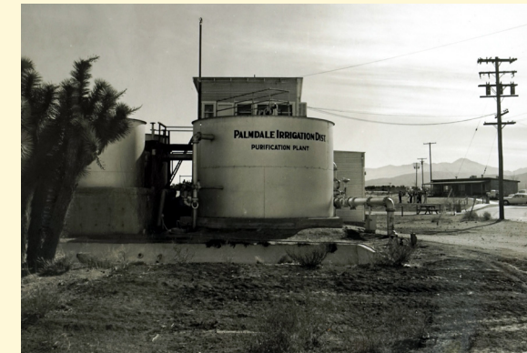
First unit of the District's water treatment facility. It was unique because it was the only plant in Southern California for domestic service except for Colorado River Works. (1955)
