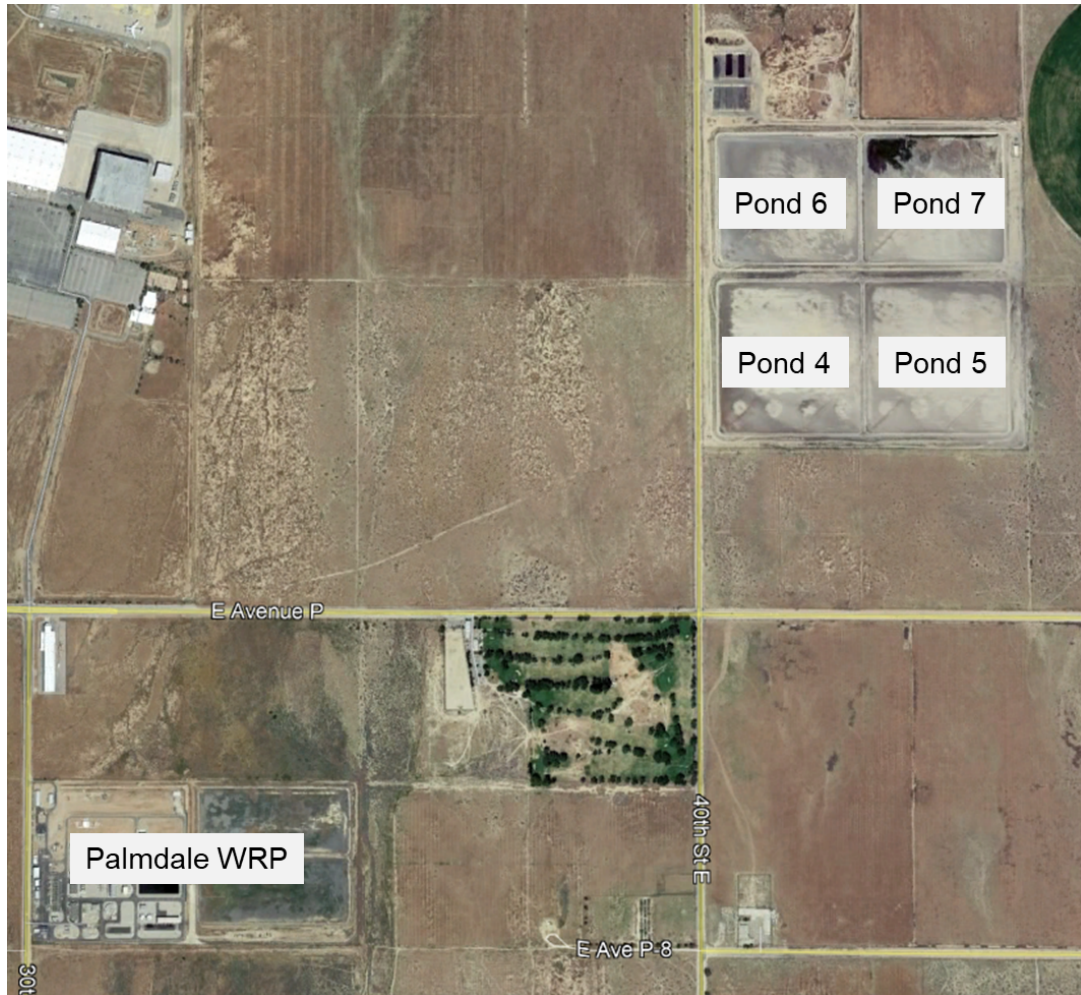
Figure 5: LACSD Former Oxidation Ponds
