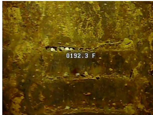
Enlarged louvered openings showing gravel envelope.
