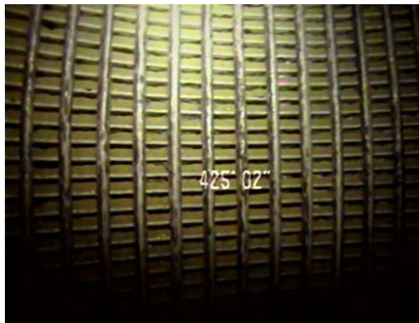
Well screen clean and giving appearance of stainless steel.
