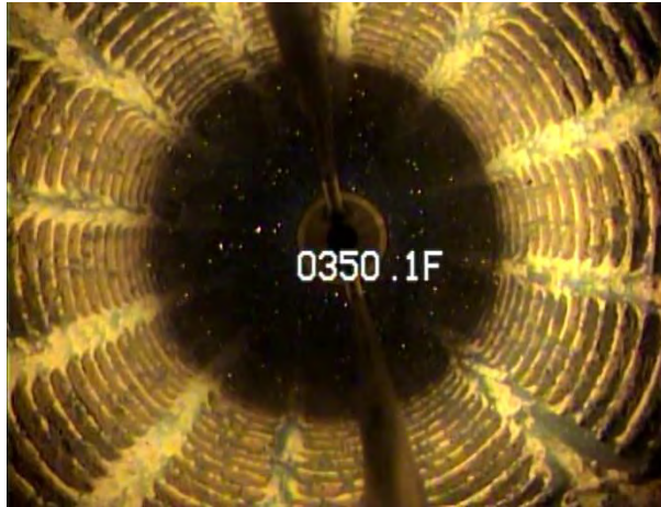
Evidence of prior bacterial growth and nodule formation.
