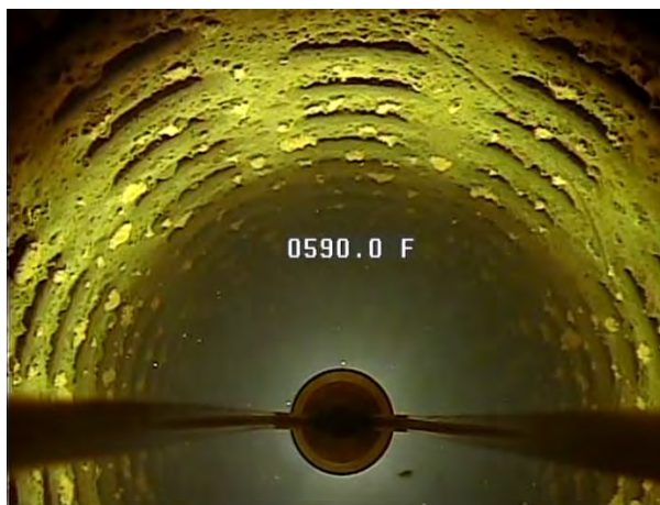
Mild encrustation and bacterial growth above 600 feet bRP.
