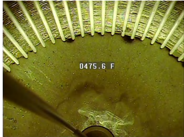
Bottom of well screen appears torn and clogged.
