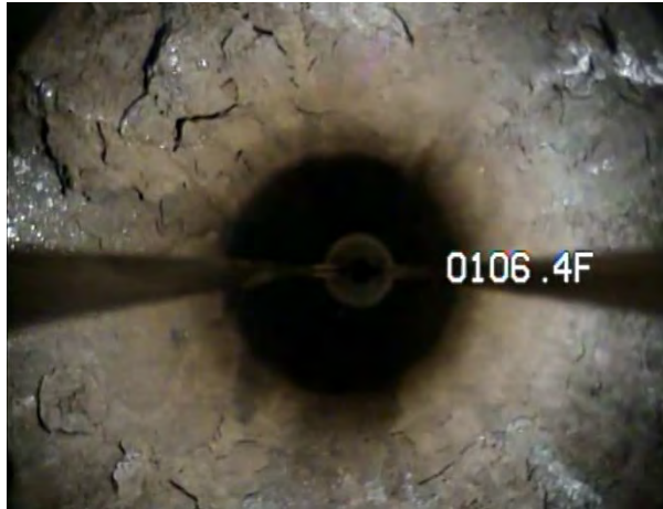
Heavy corrosion of casing immediately above water level.
