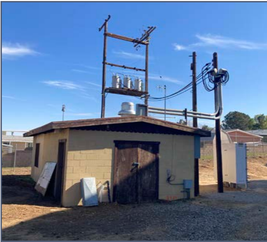
Existing pump station to be demolished
