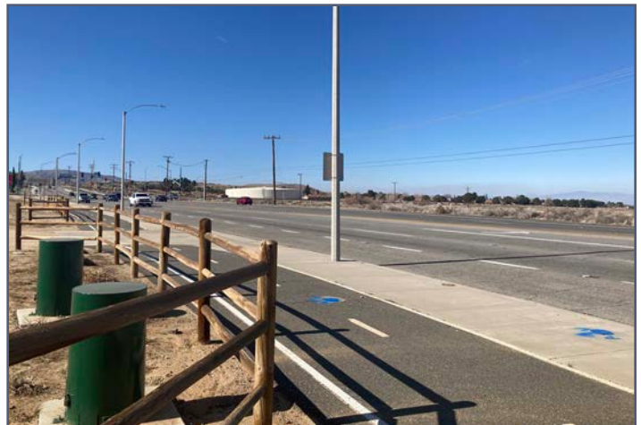
New pipeline across Avenue S
