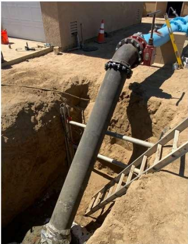
Ave P and 10 th Street Connection at Well 15
