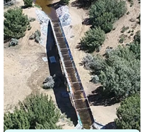
Existing Flume to be Demolished
