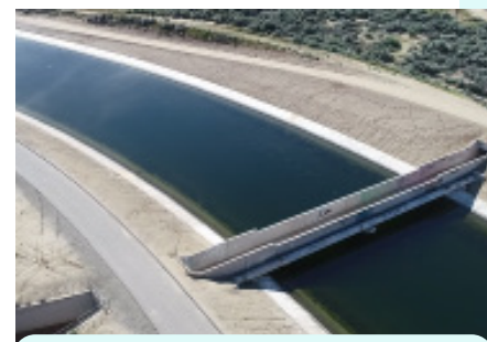
Existing Crossing of CA Aqueduct
