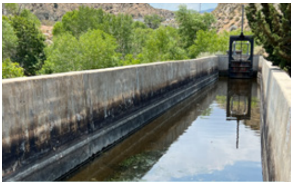
Existing Concrete Channel
