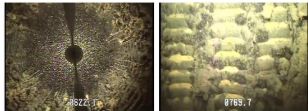
Figure 5 – Encrusting and biological material on well screen.
