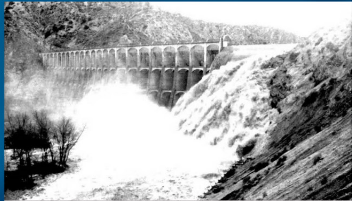
Water flowing over the Littlerock Dam's spillway before it was raised 12 feet.
