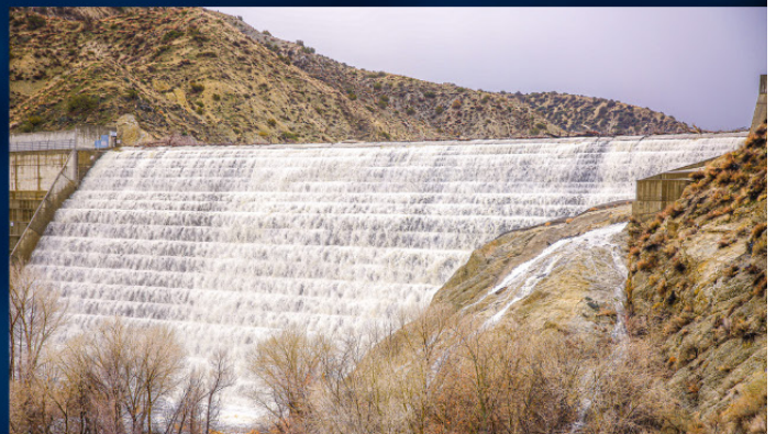
A recent photo of water flowing over the Littlerock Dam's spillway.
