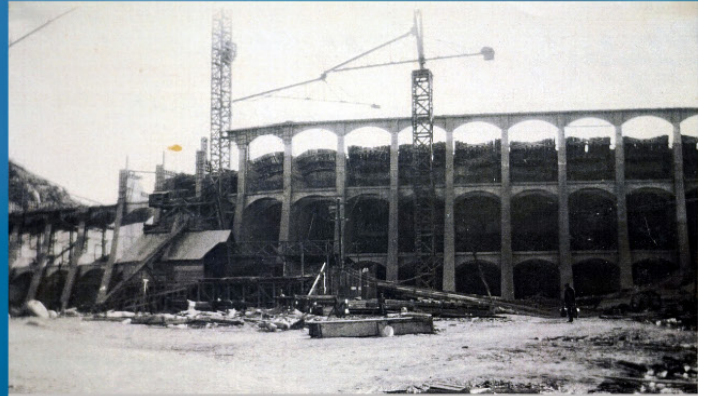
This photo shows the third stage of Littlerock Dam's construction, which began in 1922.
